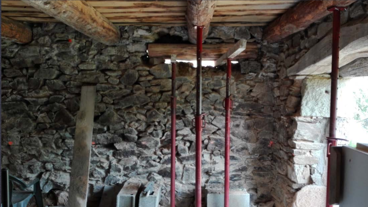
opening a door in a stone wall
