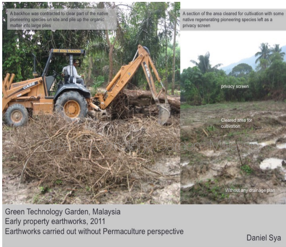
Figure 2: Earthworks during early site development of GT garden.
